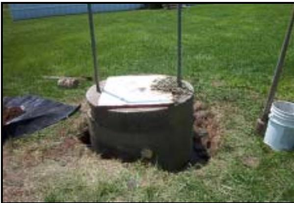
Many **older shallow wells** have **no protective** sealing or grouting.
