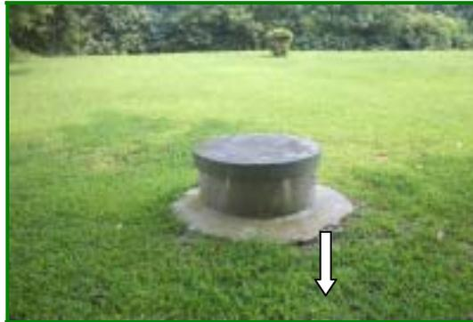
In Virginia well drillers are required to install a protective **grout (cement) down 20 feet** for shallow bored wells.
