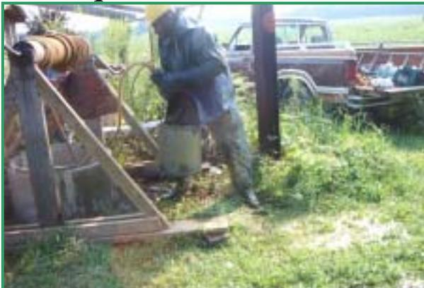
We arrived at a well site just as the crew was chlorinating and noticed that the man **was splashing most of the liquid bleach around the sides of the well**. Very little got into the well water and the water level never came up to the area that had been bleached.
