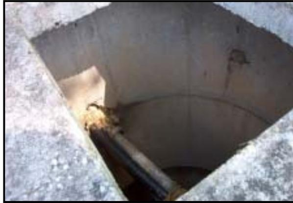
When the pipeline is installed, plumbers break a hole through the cement curb often leaving a jagged opening around the pipe where dirt can pour into the well.
