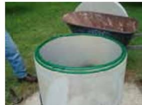
The hose doesn't need any glue but the weather stripping will need glue on the bottom. Use glue that works on cement.
